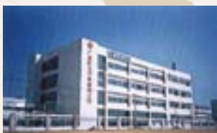
Hitachi Air Conditioning & Refrigerating, Китай
